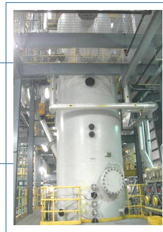
SCALABLE TO 5 MWE SKID MOUNTED TO 25 MWE+ DESIGN/BUILD
